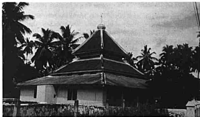
PLATE 3 Kampung Laut Mosque, Kelantan. 400-year old mosque built entirely of wood and believed to be the oldest mosque in Malaysia. The mosque with three ventilated-roof structure is distinctively Javanese in origin and it is said that the builders of this mosque were missionaries from the island of Java. (Photo: courtesy of National Museum Malaysia)
